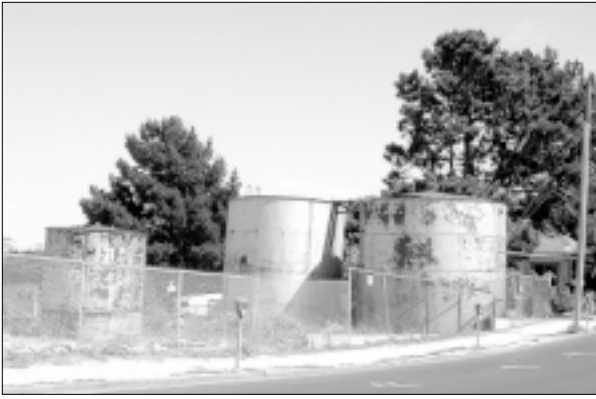
Storage tanks are representative of category “C” of Contributing properties.
