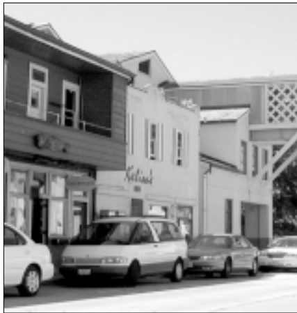
Kalisa’s is H-1 eligible. The facade has experienced alterations during its history.
