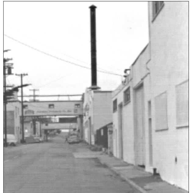
Buildings along the bay side that were traditionally a part of the cannery industry align at the sidewalk edge. Openings include large service doors. - Photography by Pat Hathaway, from the Pat Hathaway collection
